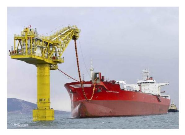
Figure E. Fixed tower single point mooring (FTSPM). Source: SBM Offshore, reproduced in Vermeulen (2011)
