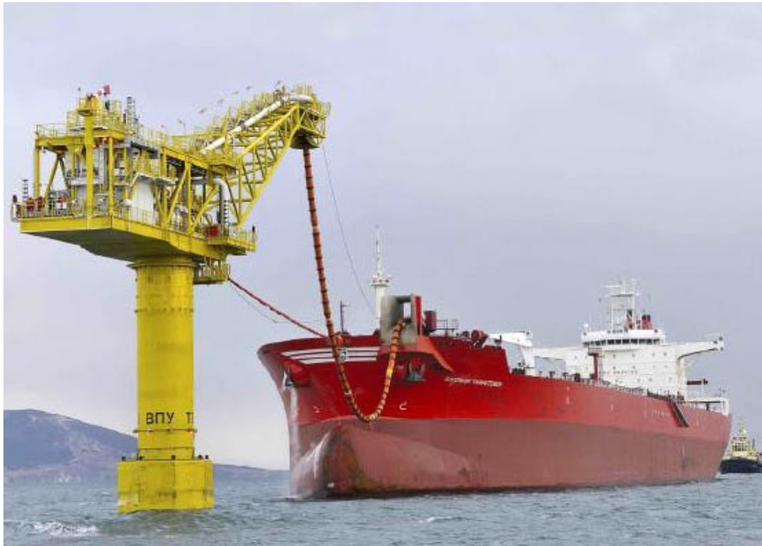
Figure E. Fixed tower single point mooring (FTSPM). Source: SBM Offshore, reproduced in Vermeulen (2011)
