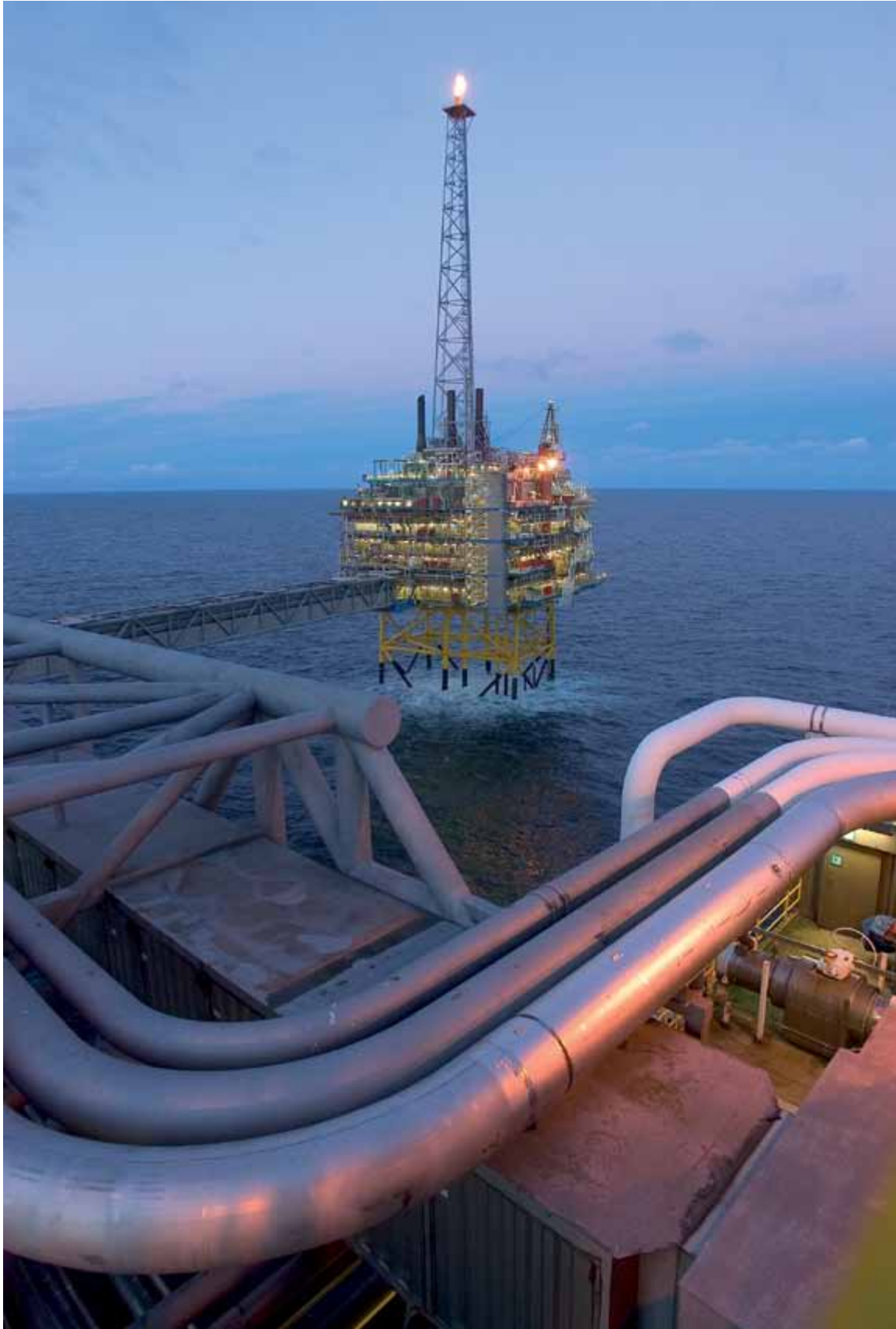
Part of the Sleipner Field CCS infrastructure, offshore Norway. Courtesy of StatoilHydro.
