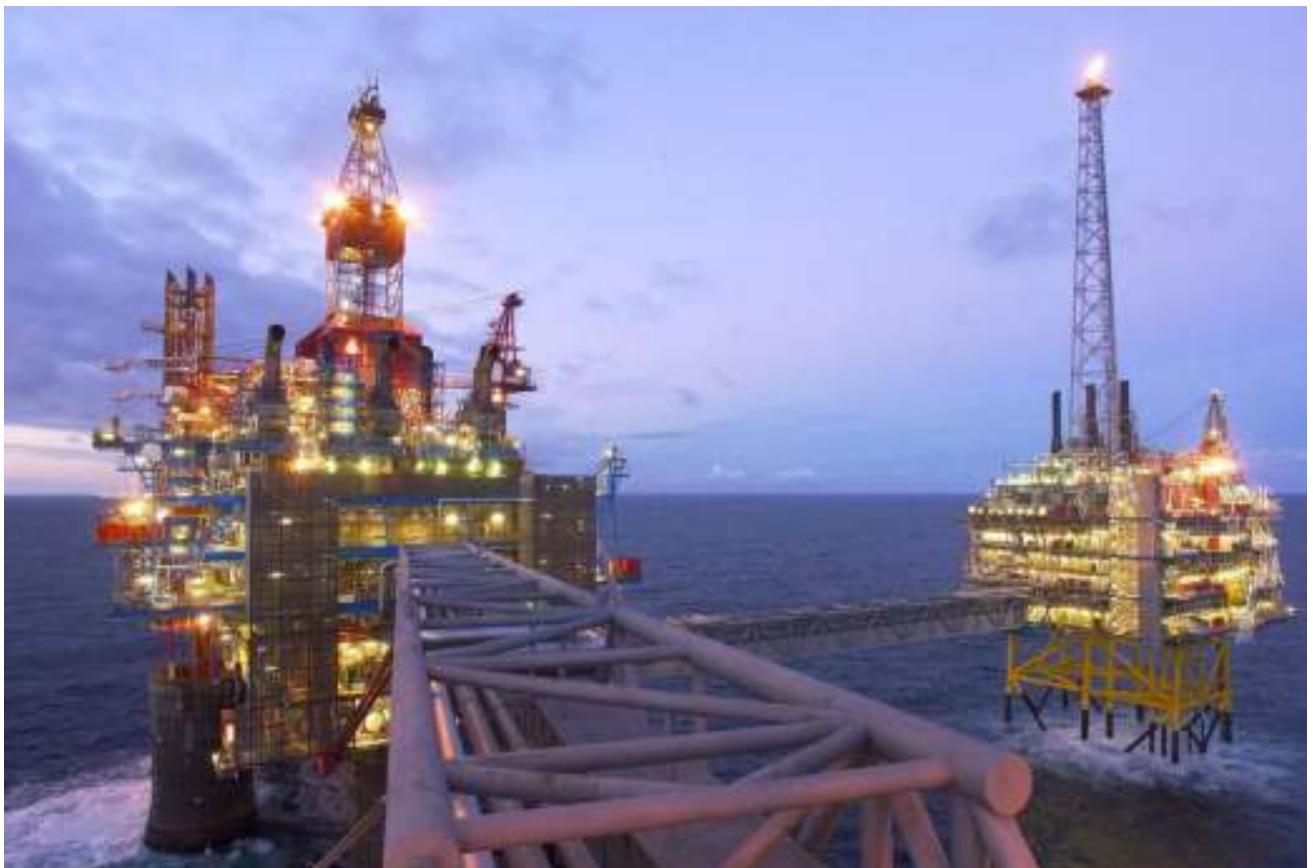
The Sleipner gas extraction platform in the North Sea where Norway's Statoil has been capturing and storing CO 2 since 1996 Photo: © Dag Myrestrand / Statoil
